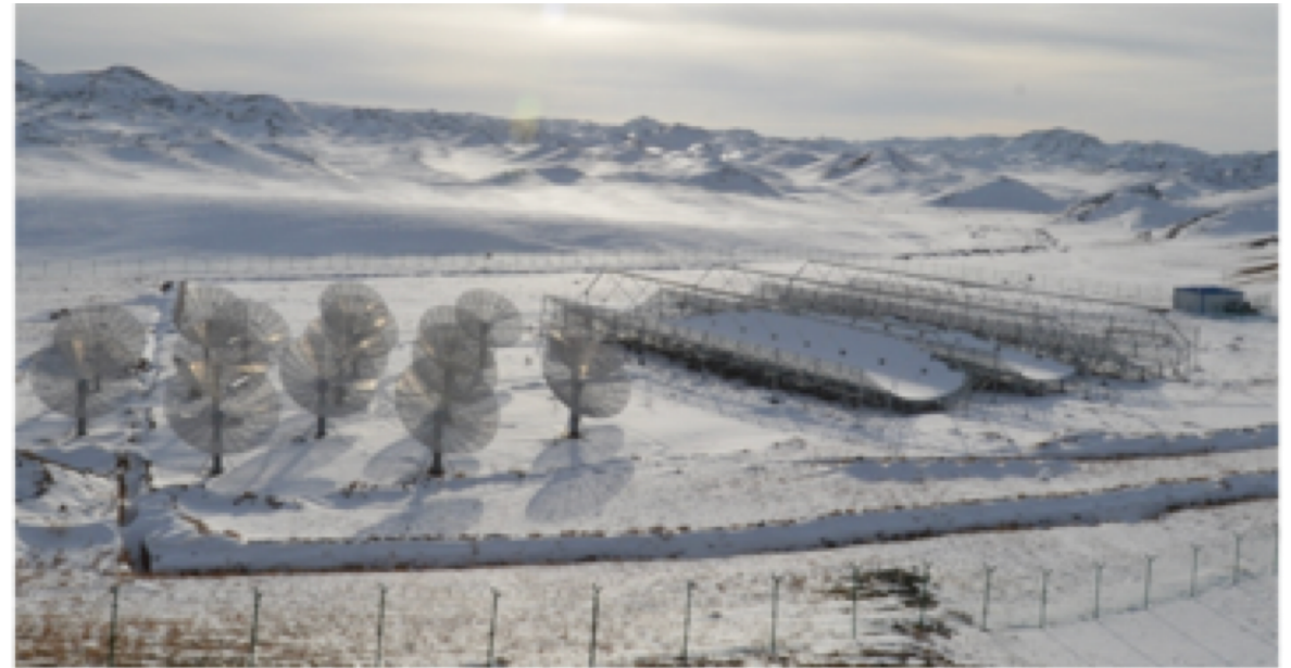
Tianlai Telescope. Credit: NAOC
