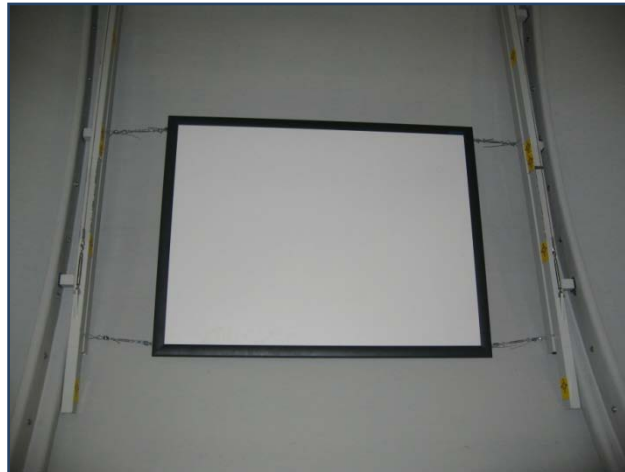
Fig. 4.13: Flat screen mounted inside the dome
